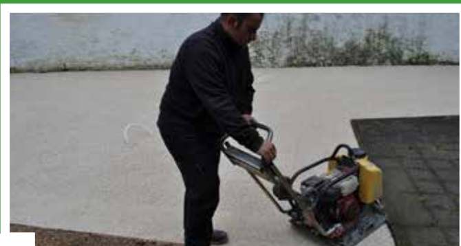
GRAVEL MANUAL COMPACTION
